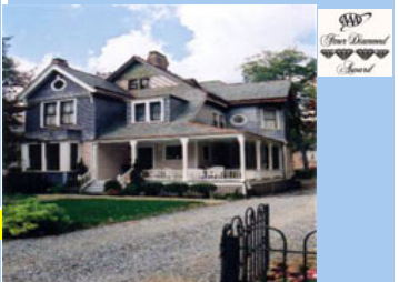
Mc Ninch House
